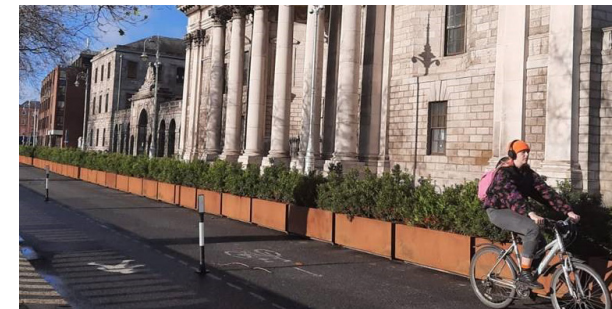
Figure 14.1 – Liffey Cycle Route at Inns Quay/Four Courts
